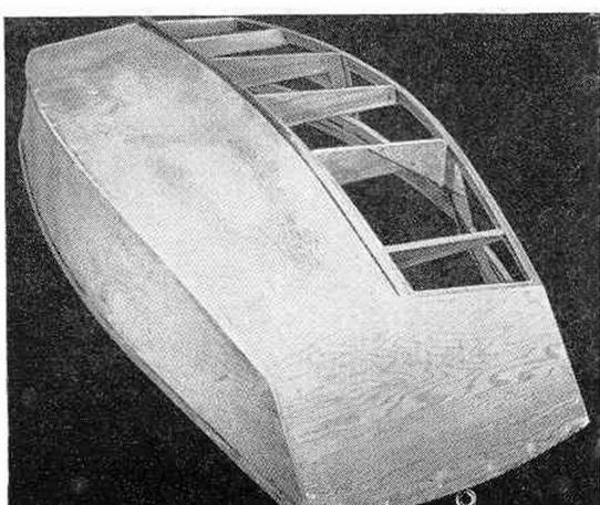
Fair the exposed edges of the plywood into the curve of the bottom and sides. Cut, fit and join the side planking, using the same material and method of fastening. Fair the edges of the plywood to the angle of the frames. At this point the boat can be removed from the building board.
