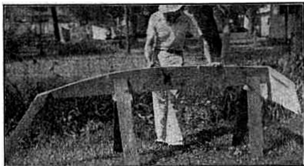
A form for the "Kingfisher" is here set up and is ready for construction work.
