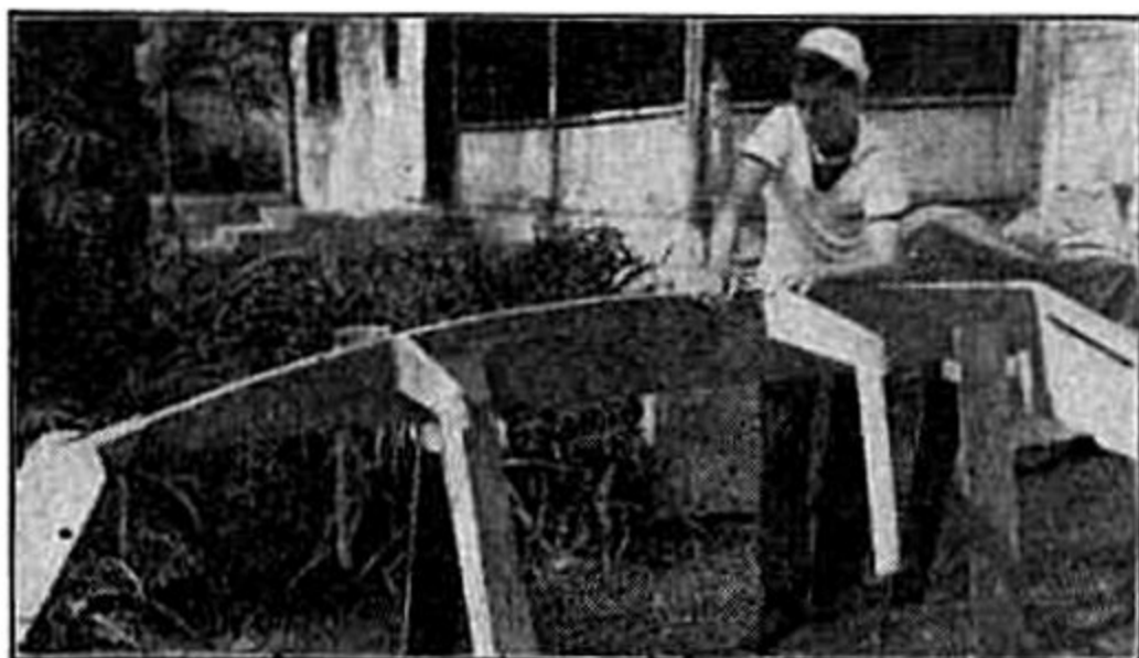
Putting the mould frames into place.
