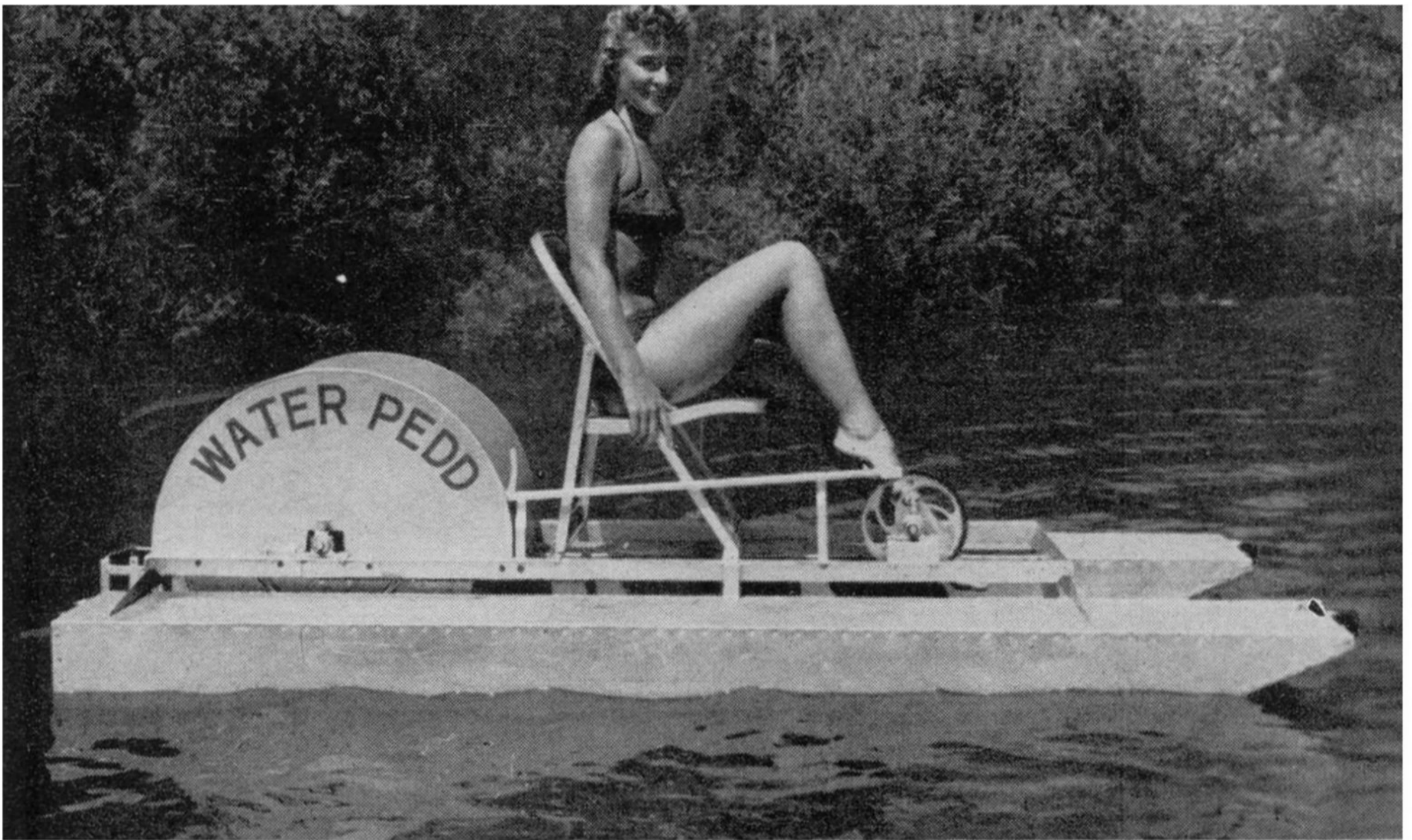
Considerable overhang at the bow ends of the pontoons, and shoal draft of this stable paddle boat permit navigating shallow streams and lakes and easy launching and boarding whether from beach or dock
