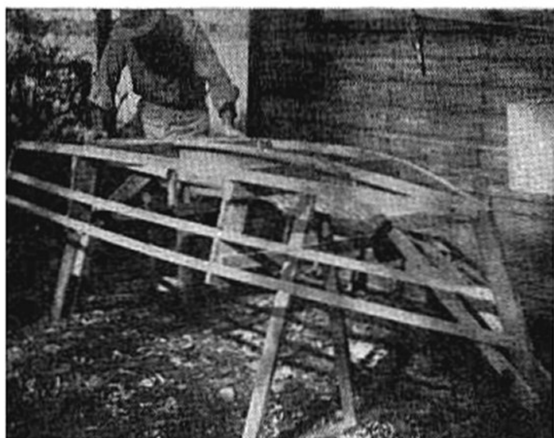
Framework completed, ready for planking.
